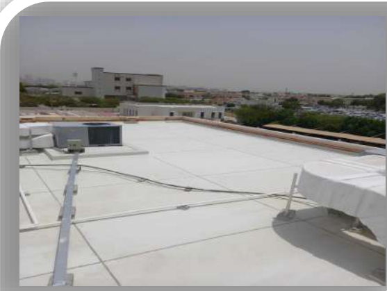
5. Joint Sealant with top coat
