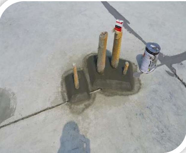
8. Finished Skirting by Pipe
