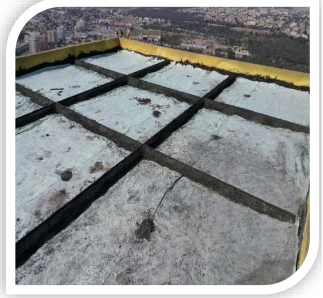
2. Geotextile & Slope
